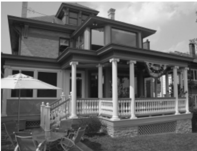
The porch addition that won a regional CotY award in the Residential Exterior Over $100,000 category for Kessler Construction Services fit seamlessly with the architectural style of the 1910 home.
