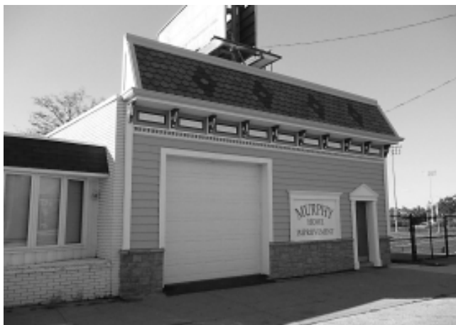
Murphy Home Improvement won local, regional, and national CotY recognition for the exterior remodel of the firm's own building.
